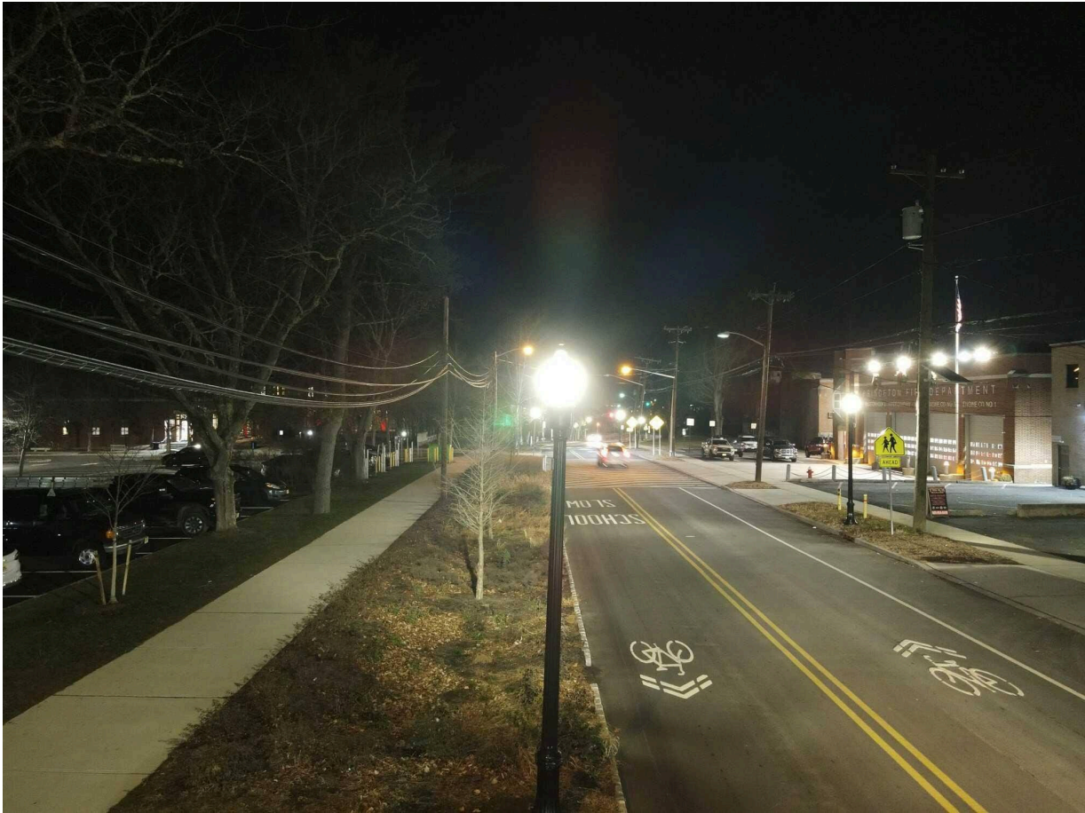
Photo taken horizontally, at the exact same height as the luminaire. Notice the excessive glare and light trespass. This is technically referred to as a 90-degree light-emission angle (0 is toward the nadir, 90 is horizontal, 180 is zenith).
