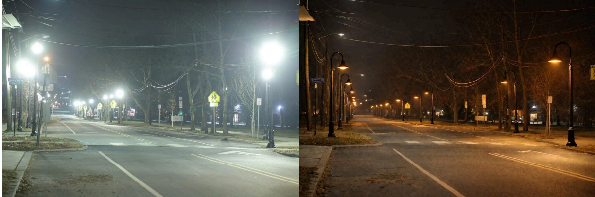
A realistic simulation of Witherspoon street demonstrating the effect of the proposed retrofit from the current fixtures (left) to the Epic Medium fixture, full cutoff, 2700K (right, simulated) . This proposed retrofit would achieve zero uplight, i.e., a BUG rating if U=0 . The pendants could also be turned outward, toward the sidewalk. Illumination levels on the sidewalk would be perfectly consistent with Princeton's municipal code.
