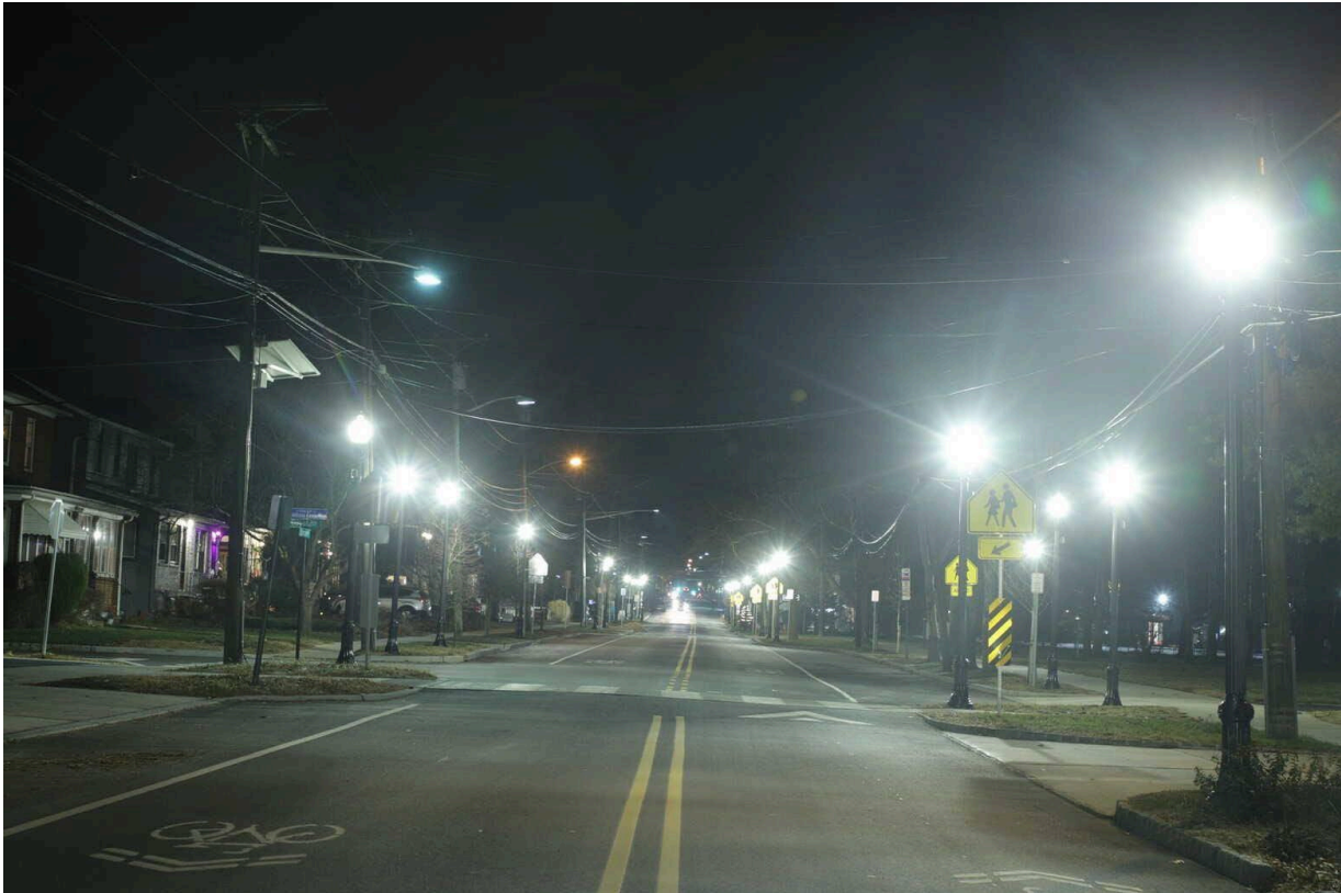
Witherspoon Street view showing everything: strong blue glare from the new fixtures; flathead halide cobrahead streetlights “overshadowed” by the new lights; one older sodium cobrahead with an orange color representing the ~2000K amber color. The glare dominates the view, reducing visibility of drivers before reaching the pedestrian crossing. This is a textbook example of more lights not improving the overall visibility.
