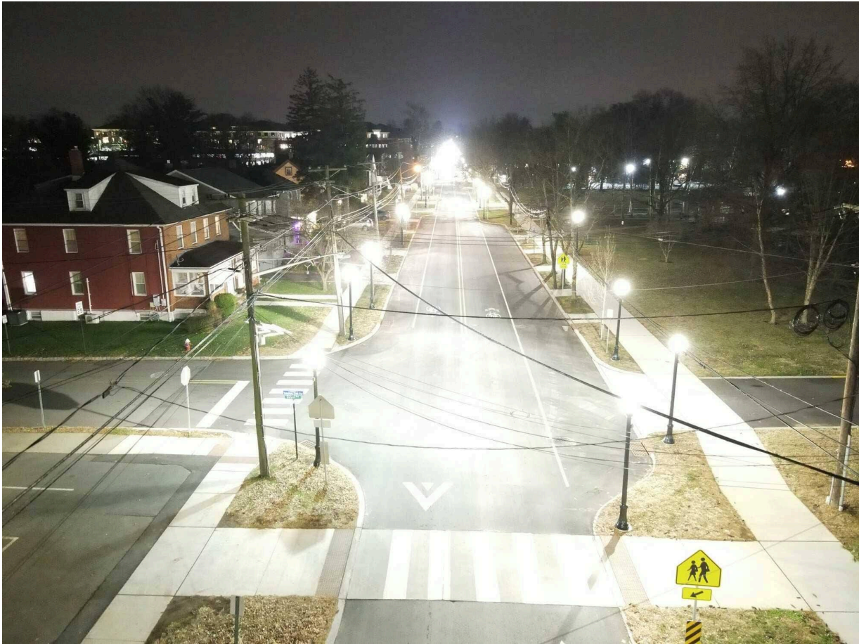
Witherspoon Street from about 10m above ground. The image demonstrates overlighting and harsh lighting with a strong glare and an upright component.
