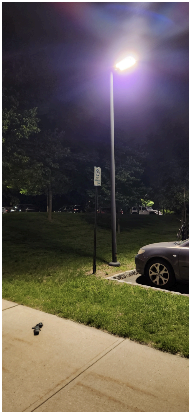
(D) Dinky parking lot walkway, seriously overlit, 4.55 FC measured.
