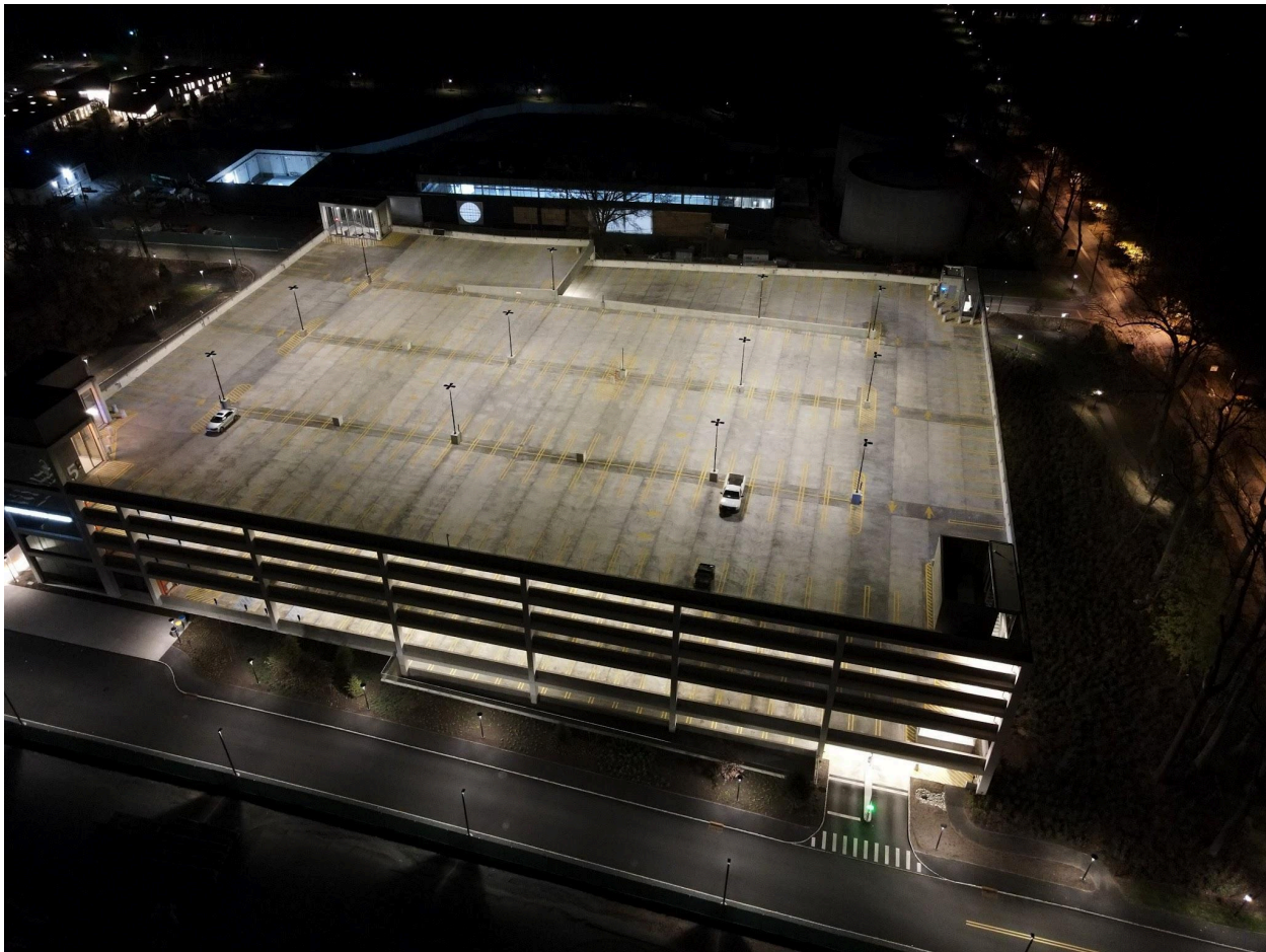
Stadium Drive Garage. Note the very high illuminance with respect to e.g., the pedestrian walkways and the adjacent Faculty Road. The direct illuminance is 2.3 FC. This is independent of the high albedo of the garage.
