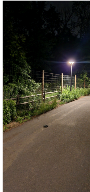
(B) cont. 3.63 FC beneath pole, 0.59 FC between poles, respectively. (Desired: 0.3 FC).
