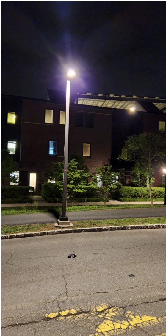
(A) These are low post LEDs with ~3000K light, 2.92 FC directly beneath pole, 1.6 FC between poles at the center of the street. (Desired value 0.3 FC).
