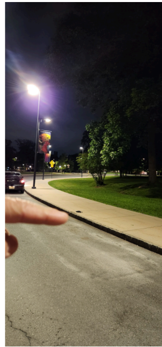
(A) Shoebox LEDs on high poles. Generally overlit, and the lighting is homogenous due to the high poles. 3.59 FC directly beneath the pole and 2.15 FC between the poles, respectively. (Desired value 0.3 FC).
