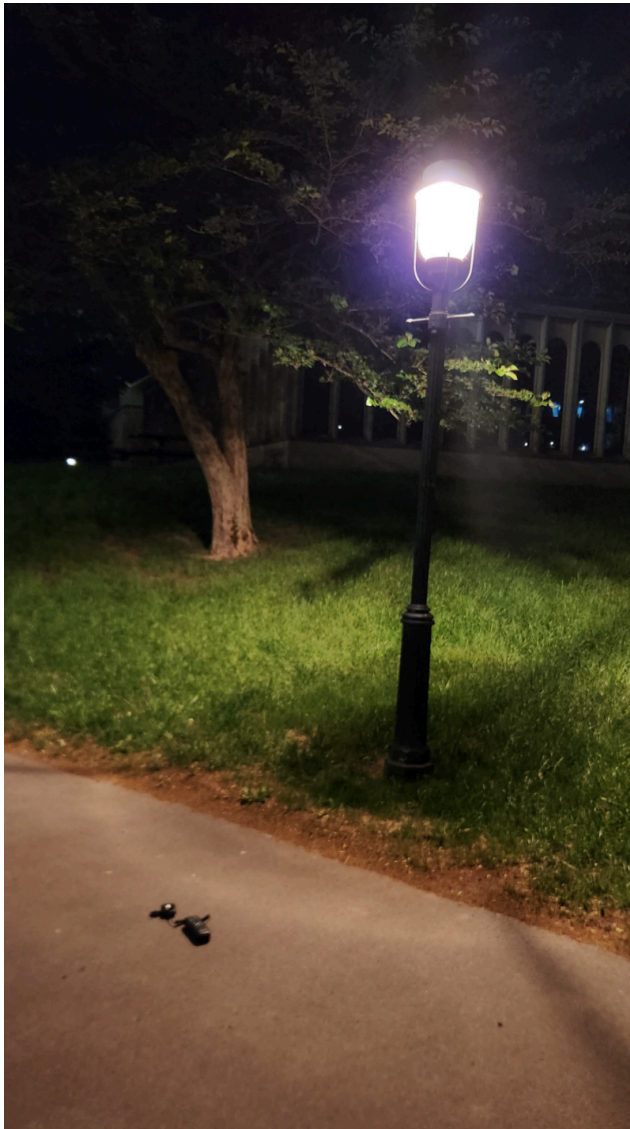
(A) cont. Southside of Peyton Hall, directly beneath the lamp. Measurement of 3.46 FC (target 0.3 FC).
