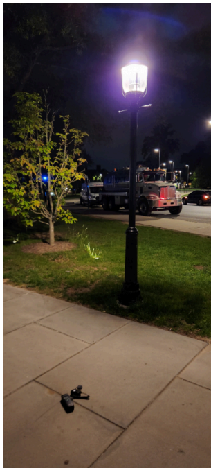
(B) Overall, slightly overlit area. 2.6 FC directly beneath the pole, 0.47 FC between the poles, respectively. (Desired 0.3 FC).
