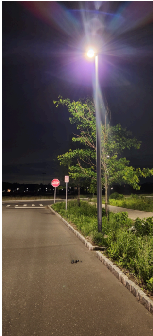
(E) The walkway is excessively illuminated, with both roadway and sidewalk fixtures operating at light levels far higher than necessary, 3.47 FC beneath the pole and 1.66 FC between poles, respectively. (Desired 0.3 FC).
