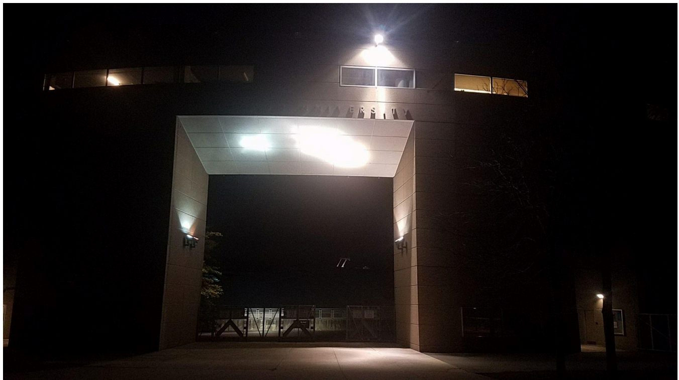
Archway lights of the stadium. The upward-oriented lights are bright, and a fraction of the light misses the building, shining up in the sky.
