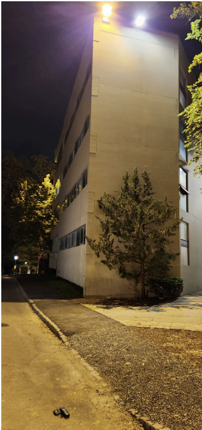
(B) Strong area lights from the top of the building, causing glare and overlighting, 4.3 FC measured. (Desired value 0.3 FC).
