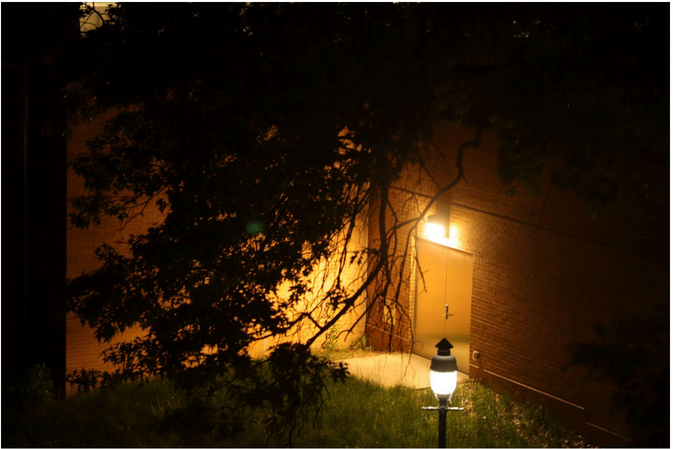
Unshielded area light next to Peyton Hall on the Lewis Library building. The light of this fixture directly shines in the Peyton telescope dome when the dome slit is open. It is also excessively bright, causing glare for pedestrians.
