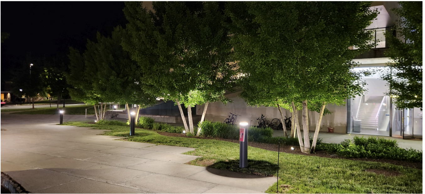
(C) Sharp white glare from a large cluster of unshielded bollards shining directly in the eye, next to Princeton Station.
