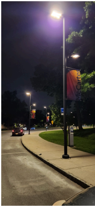
(A) Shoebox LEDs on high poles. Generally overlit, and the lighting is homogenous due to the high poles. 3.59 FC directly beneath the pole and 2.15 FC between the poles, respectively. (Desired value 0.3 FC).
