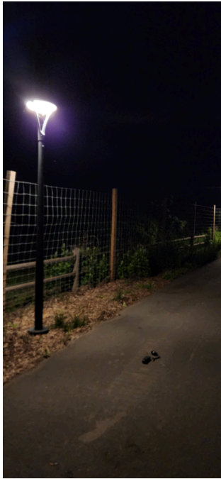
(B) cont. 3.63 FC beneath pole, 0.59 FC between poles, respectively. (Desired: 0.3 FC).
