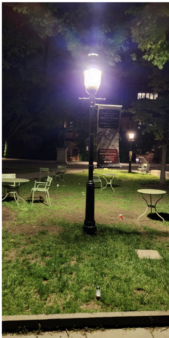
(A) cont. Penn globes, measured at 0.62 FC between poles and 2.28 FC beneath the pole, respectively. (Desired value 0.3 FC).
