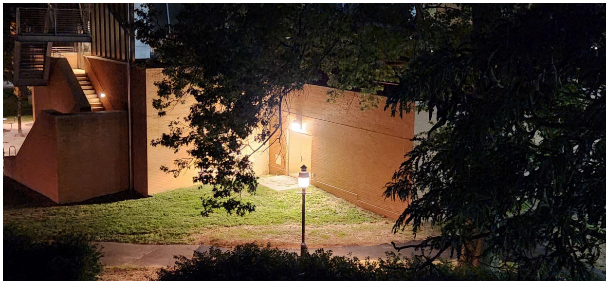
Unshielded area lights directly illuminate the roof.
