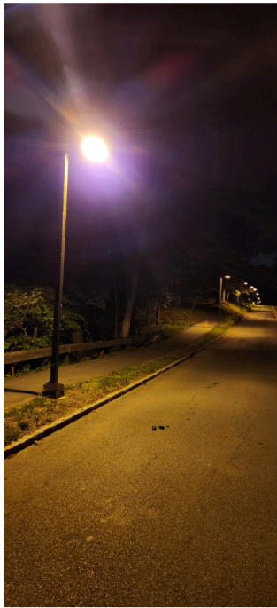
(B) Low post shoebox sodium, very well shielded, slightly overlit. One of the best lighting on campus, even though the backlight is not desirable at other parts of Faculty Rd. Closer to Broadmead. 5.15 FC directly beneath pole, 0.81 FC between poles, respectively.
